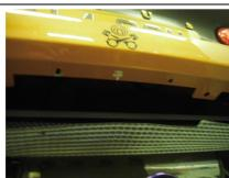
6. Existing Lotus fixing holes shown at top where M6 threaded anchor nuts have to be fitted.
