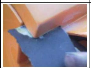
3. Sand off lip uder rear clam shell where the blanking piece was fitted.
