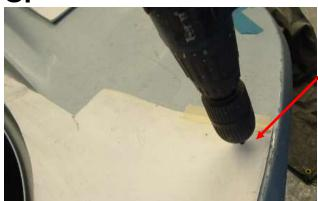
WITH A SMALL DRILL BIT (3-4mm IS IDEAL) PILOT DRILL THE FOUR MOUNTING HOLES INDICATED ON THE TEMPLATE, THEN REMOVE THE TEMPLATE AND DRILL THE HOLES OUT TO 7.5mm.
