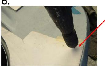
WITH A SMALL DRILL BIT (3-4mm IS IDEAL) PILOT DRILL THE FOUR MOUNTING HOLES INDICATED ON THE TEMPLATE, THEN REMOVE THE TEMPLATE AND DRILL THE HOLES OUT TO 7.5mm. Remove the paper template
